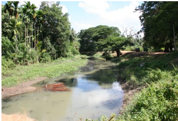
Figure 10. An ancient feeder canal close to the modern one in figure 9, with a single bank that trap the local inflow and slow velocity as it is a contour canal that retain a large command area.
