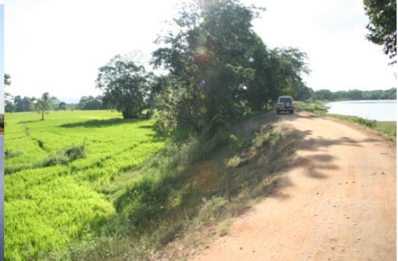
Figure 6. Embankment of a tank
